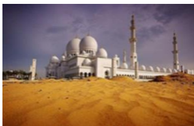
Fig. (13) The mosque rises 9.5 m above the ground level
